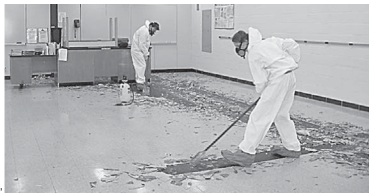
Asbestos-containing floor was properly removed from a JHS classroom as part of the renovation plan.
